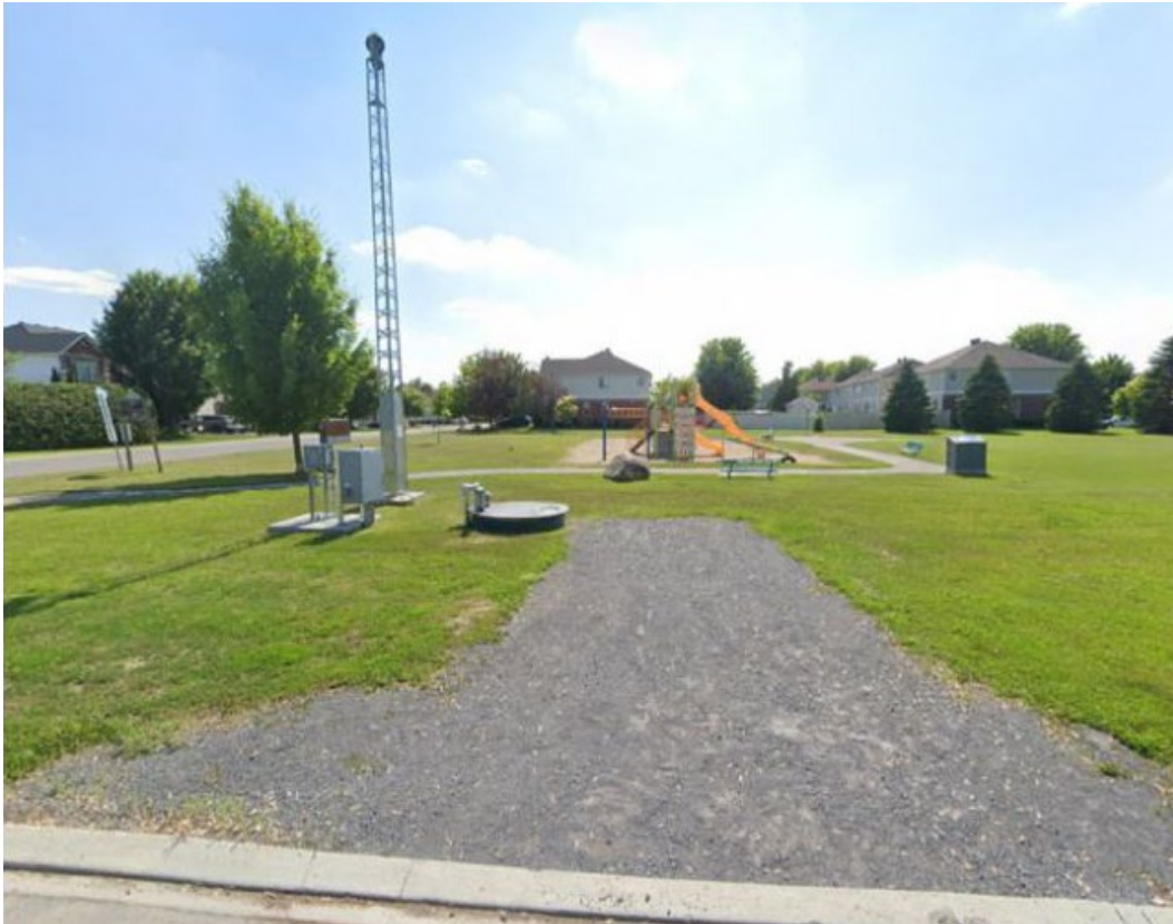
FIGURE 4 - REPRESENTATIVE EXAMPLE OF BELOW GROUND PUMPING STATION COMPONENTS AND ABOVEGROUND PANEL
